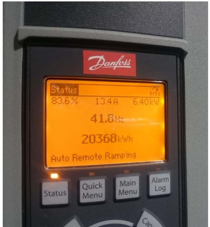
Pump Speed and Consumption after VSD Installation
